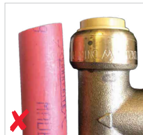
Pipe has not been cut square
